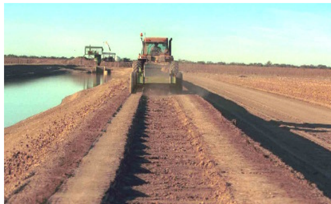
Figure 3. Improvement works on channel banks, NSW.
