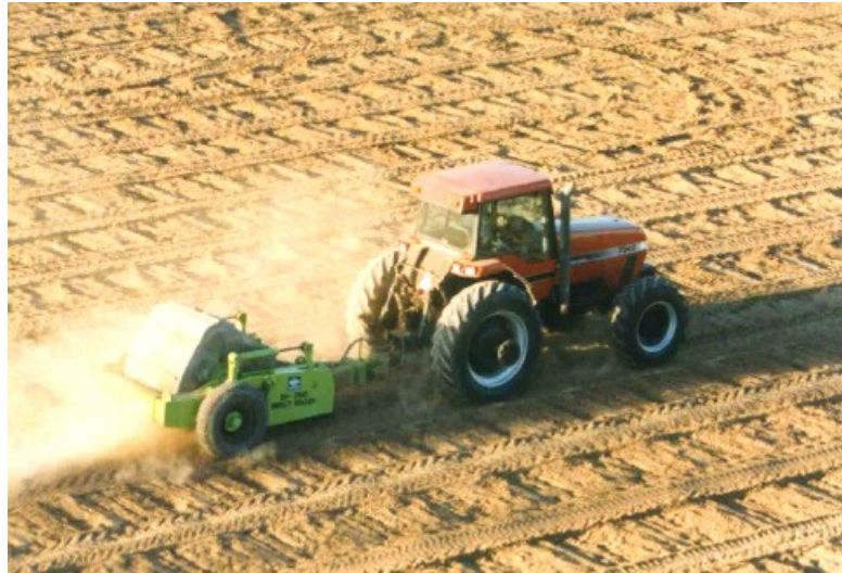
Figure 2. Impact rolling water storage base, NSW.
